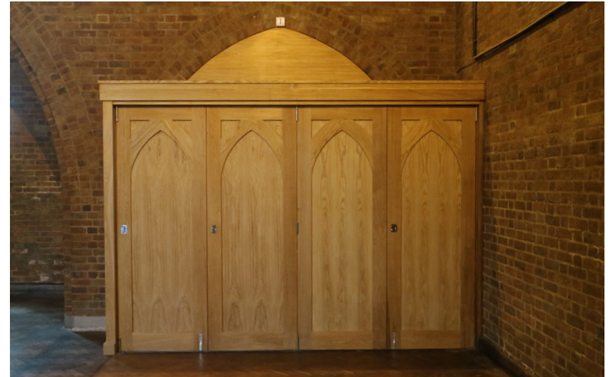
View of oak infill to arch and concealed tea station within oak cupboard
