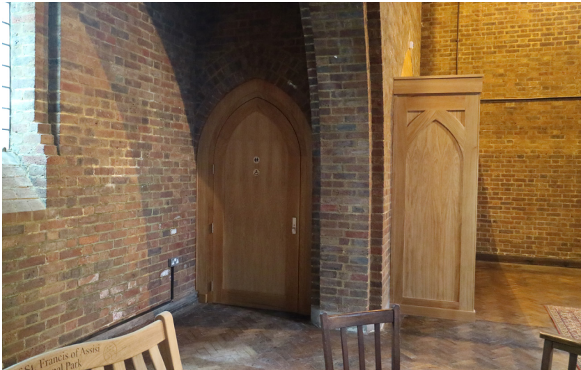
Infill to arcade with new oak door to WC and tea station cupboard on right
