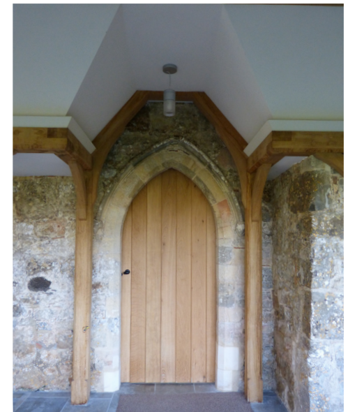
Reopened doorway from pentice to nave
