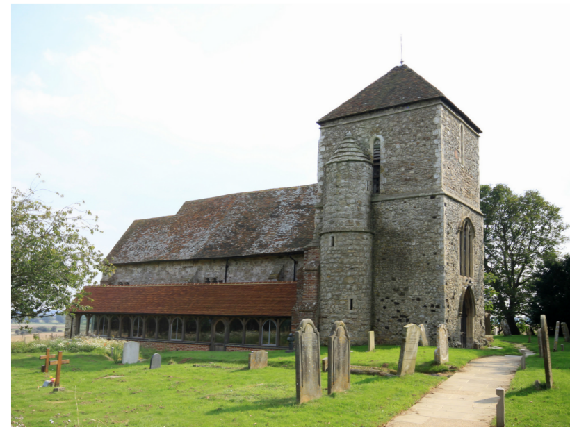
View of church with new 'pentice' extension
