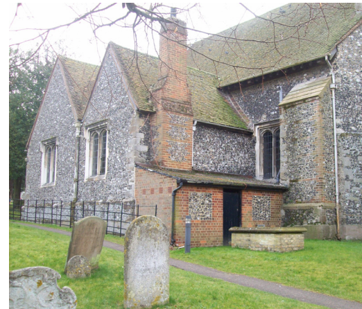
View of church from the north showing the north aisle & boiler room before reordering
