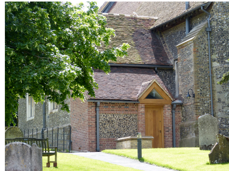
View of new entrance porch adjacent to north aisle
