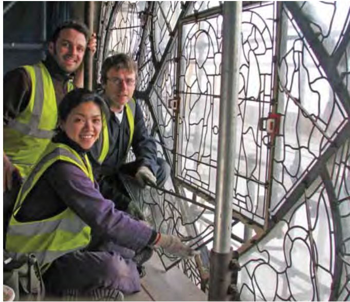
The stained glass studio team fitting a ferramenta window frame at the Cathedral.
