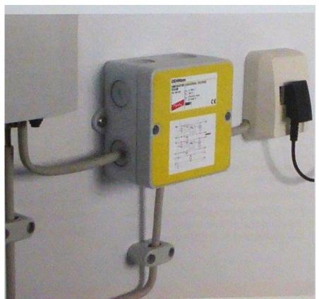
then they should still be fitted with surge protection with an earth connect but there would be no cable to a master socket.
